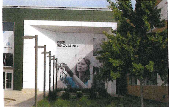
RESEARCH AND DEVELOPMENT OFFICES AND LABORATORIES
